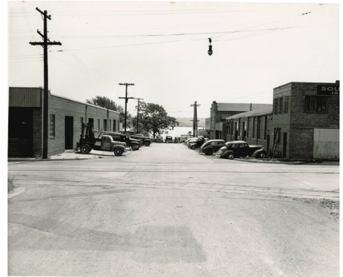
Buildings at #1 Duke Street in the 1940s.
